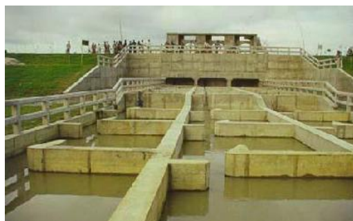
Photo 6-3: Vertical slot fish pass
