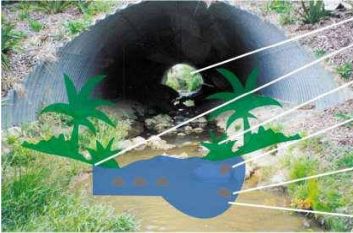
Figure 10-1: Fish friendly culvert
